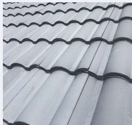
Does your roof appear faded or dull? Environmental fallout such as salt residue, dirt or dust deposits can cause this aesthetic change.
