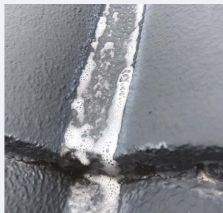
Cleaning your roof helps remove the environmental fallout.
